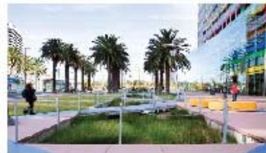
Stormwater wetland in urban plaza, Melbourne, Australia.
