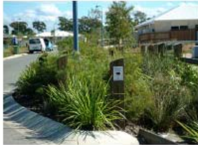
Bioretention basin in residential development, Australia
