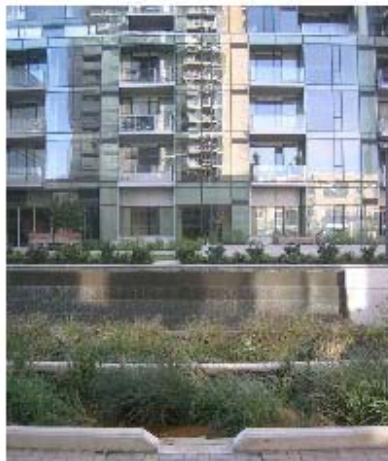
Bioretention basin in high density residential development, Portland
