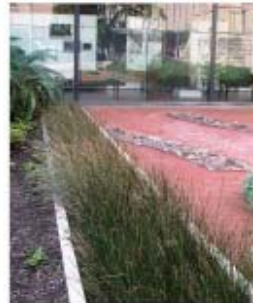
Bioretention basin in museum courtyard, Adelaide, Australia
