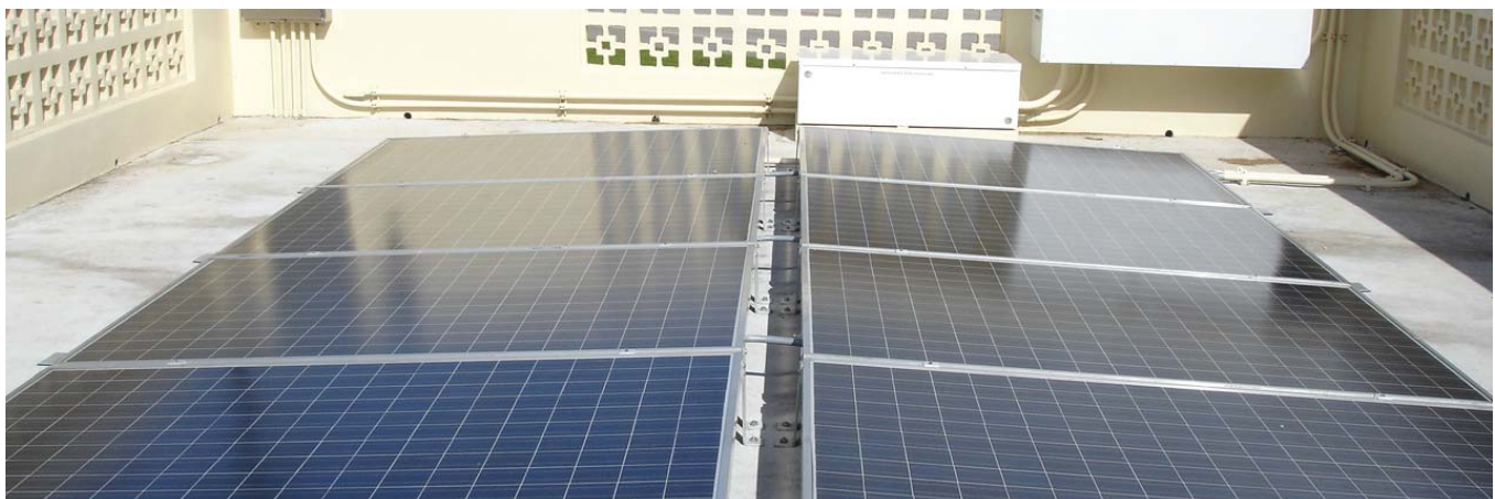
Ground mounted PV with site wall for wind protection
