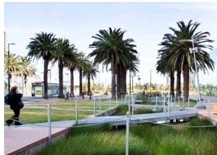
The use of Bioswales and Created Wetlands is critical to providing stormwater quality.
