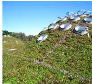
Green roof from the California Academy of Science, San Francisco, CA.
