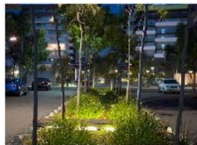
Bioretention basin in streetscape right of way, Sydney, Australia
