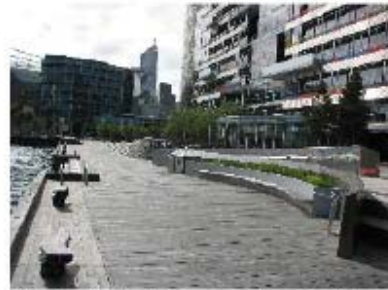
Bioretention basin in urban plaza also functioning as a bench, Melbourne, Australia
