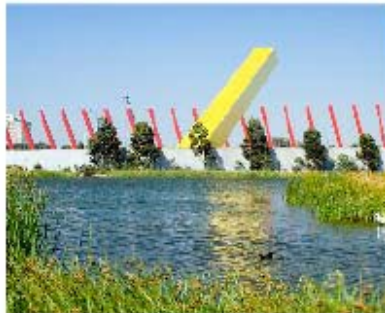
Stormwater detention pond, Melbourne, Australia.
