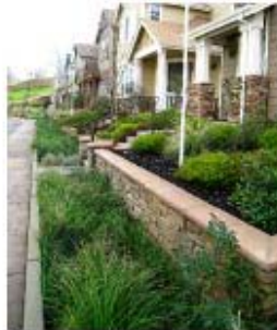
Bioretention basin in high density residential development, Clayton, CA
