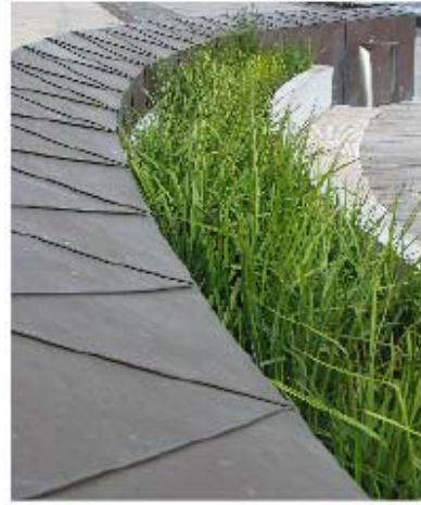
Bioretention basin in urban plaza also functioning as a bench, Melbourne, Australia
